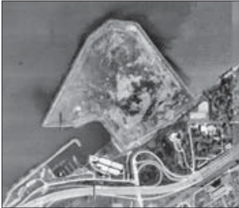
Perimeter dike, bulkheaded and ringed with boulders, confines contaminated soils
