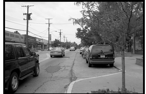
Bulbouts help moderate traffic along Lee Road in Cleveland Heights.
