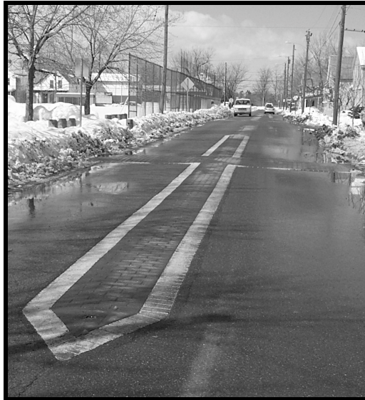
Narrowing lanes to slow traffic: Burlington, VT, uses paint and brick-patterned asphalt to create the appearance of narrower lanes near a school.
