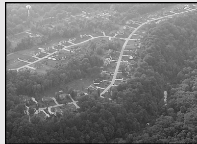
Homes encroaching on a river corridor in Lake County.
