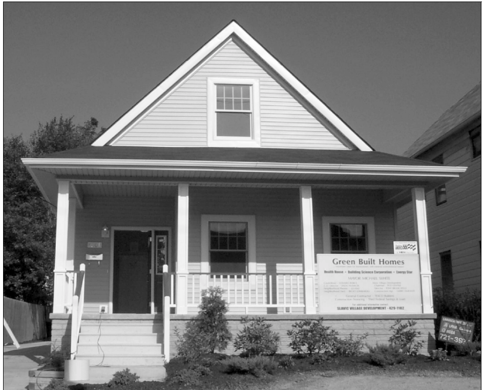
Prototype green house: The GreenBuilt home on Cleveland's east side provides affordable comfort while being easy on the environment.
