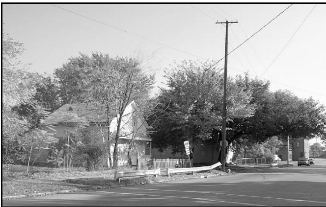
Development site: A site on W. 58th Street composed of mostly vacant lots will soon have up to 20 new homes.
