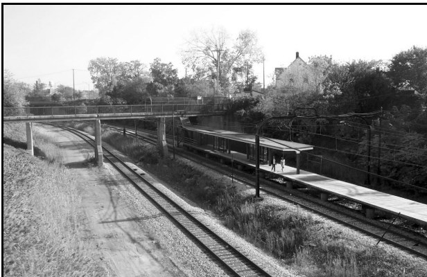
Neglected asset: The existing W. 65th Rapid station.
